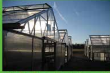
TRANSLUCENT ROOFING AND WALL PROJECTS
