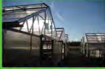
TRANSLUCENT ROOFING & END WALL PROJECTS
